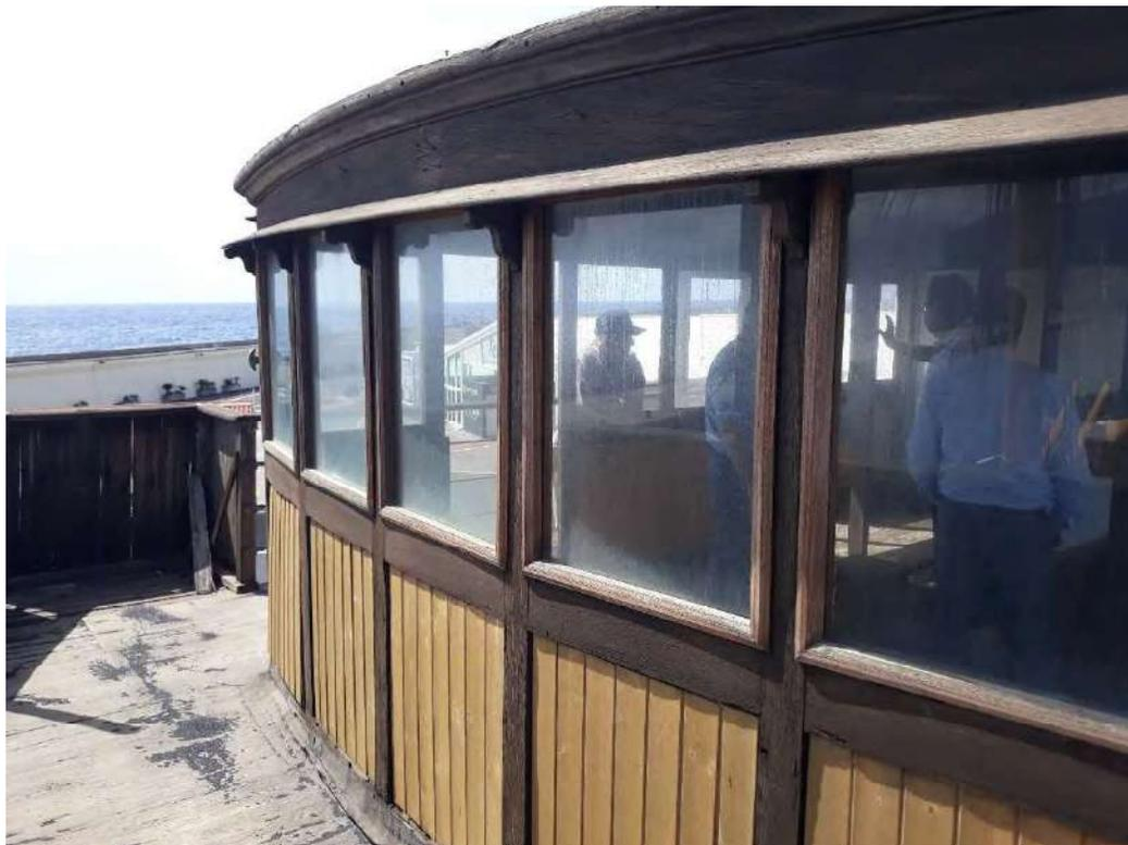
CUBIERTA, FRENTE DEL PUENTE Y BARNADILLA A REMOVER. POR SU ALTO DETERIORO
